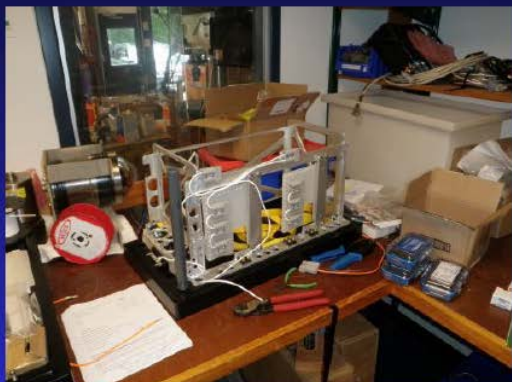
Battery chassis during assembly
